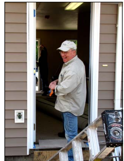
David Marquis at a recent Habitat for Humanity build.
